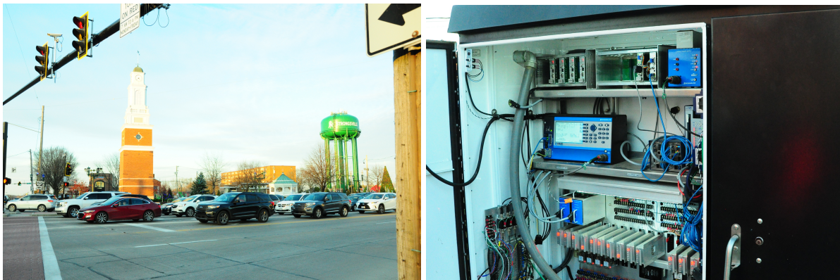
(a) Queued traffic at the intersection of Pearl Road (US 42) and Royalton Road (SR 82), during the evening rush hour at 5 pm. (b) Inside a signal controller cabinet installed at the intersection, including an Econolite Cobalt controller on the second row.
